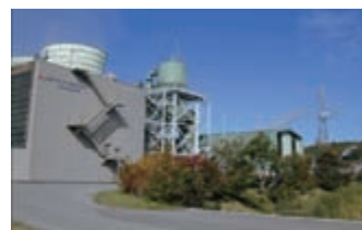
Ohnuma Geothermal Power Plant (9.5MW)
