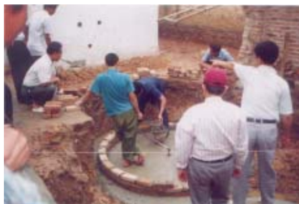
Construction of Biogas plant
