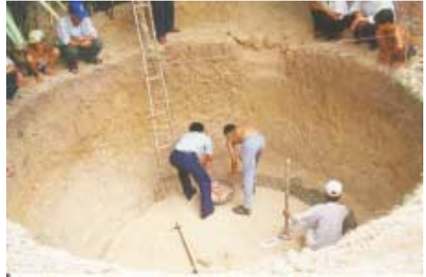
Construction of Biogas Plant
