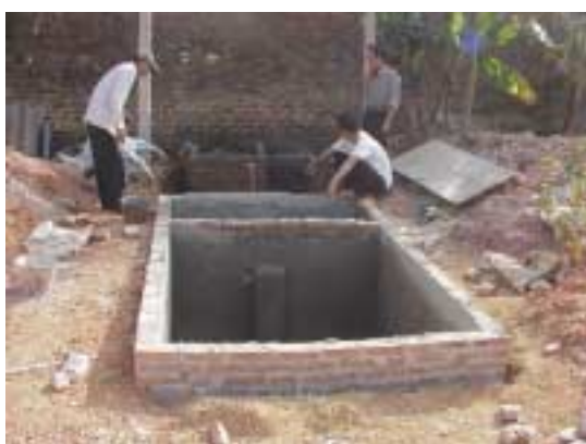
Installing a Biogas Chamber
