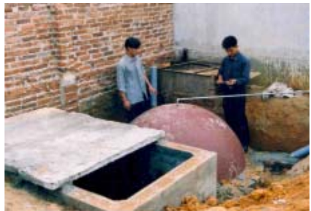
Installing a biogas plant
