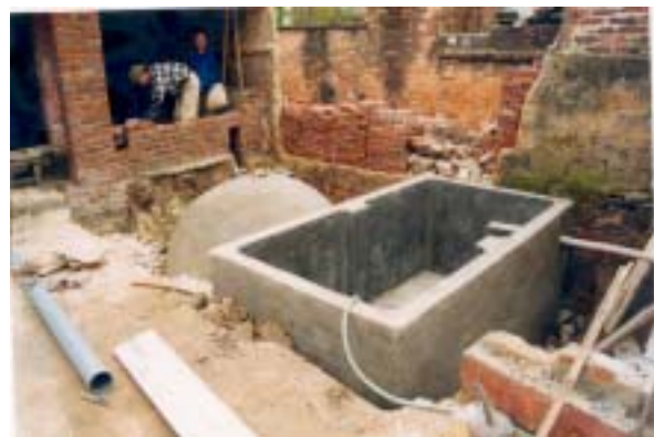
Construction of biogas plant
