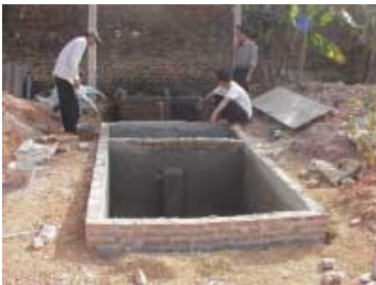
Installing a Biogas Chamber
