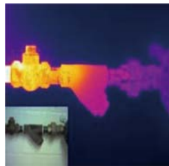
Figure 3. IR thermographic image of an operating steam trap.
