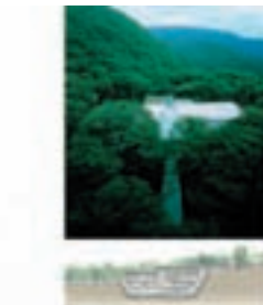
Cross section: The hemispherical substructure was designed to avoid interrupting the flow of groundwater.
