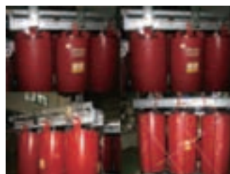
DISTRIBUTION & POWER TRANSFORMER 3 \phi 60HZ 22.8/11.4KV-380Y/220V 2500KVA 3 \phi 60HZ 22.8/11.4KV-380Y/220V 2000KVA 3 \phi 60HZ 22.8/11.4KV-380Y/220V 1500KVA 3 \phi 60HZ 22.8/11.4KV-380Y/220V 1250KVA
