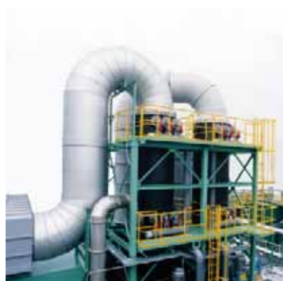
Odour control device for rendering plant
