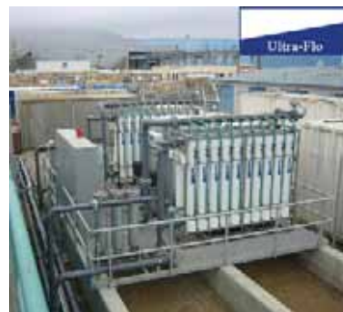
2 x M-20 Ultra-Flo® System (Installed at oil refinery in Baku, Azerbaijan for sewage treatment)
