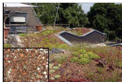
ZinCo green roof using Zupermix as growth media and Growth Media, Zupermix
