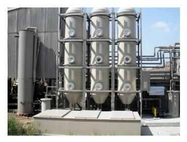
Figure 3. Farm-scale biogas biofilter system established in 2009 (for 9,000-head pig farm). Source: Su J.J.
