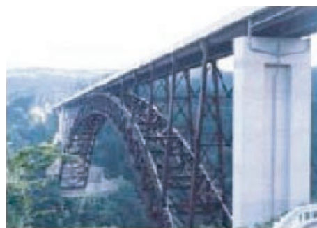
Oku-Aso Bridge constructed by using weathering steel
