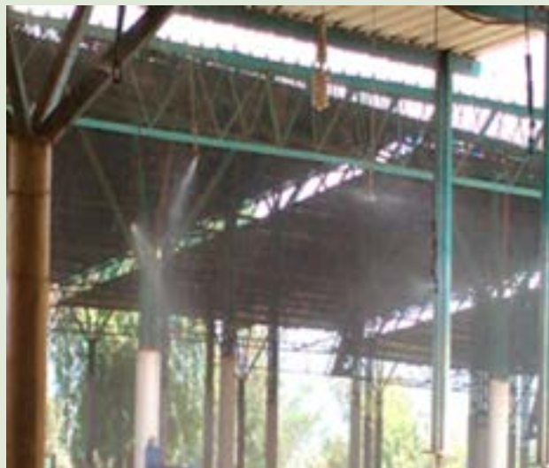
FOGGING SYSTEM IN A DAIRY SHED.
