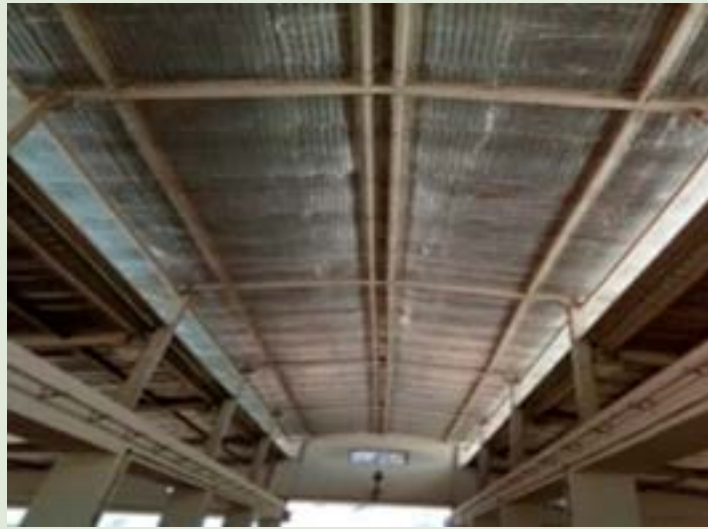
WIDE SPANNED RIDGED ROOF.
